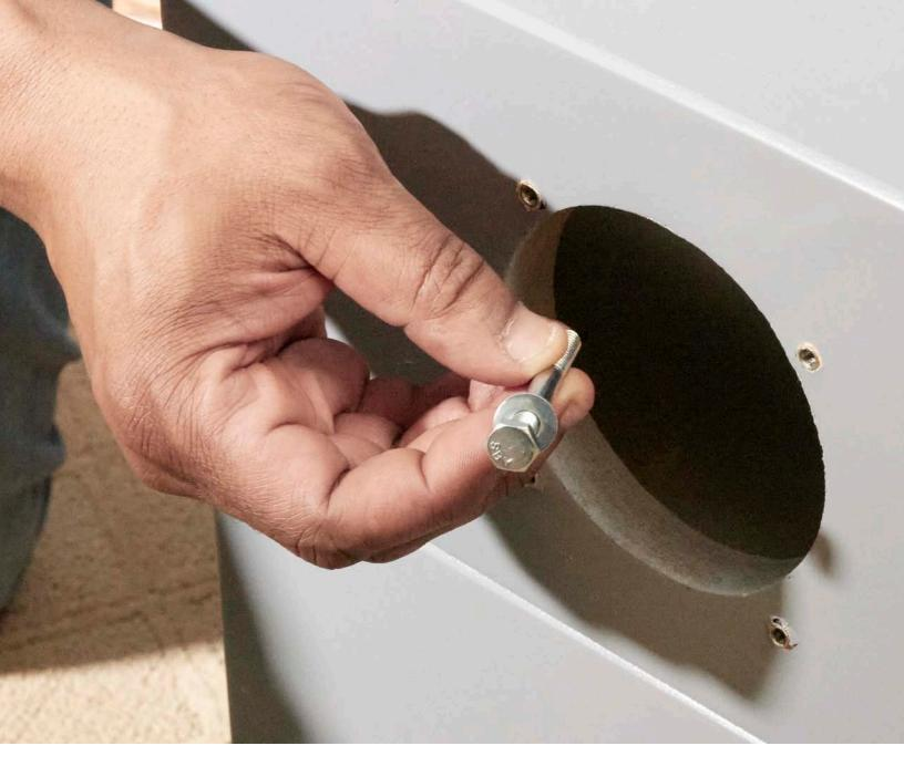
12. Locate the four drilled holes inside the bottom of the next stacked module.
