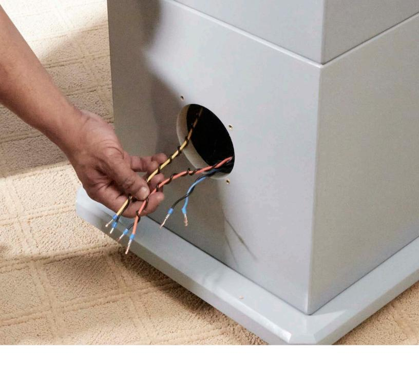
21. Fish the two upper twisted pairs of wires of each stacked module all the way down through all the modules' top and bottom holes, to inside the base woofer module, and out the back hole.
