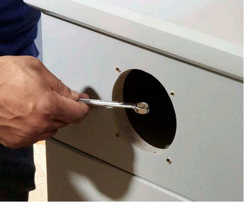
19. Use the provided 7/16" box wrench to tighten the bolts into the threaded nut inserts in the cap platform.
