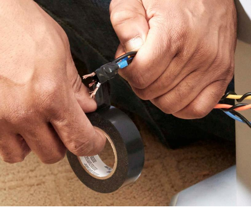
22. Using the provided electrical tape, wrap all three twisted pairs of wires together.
